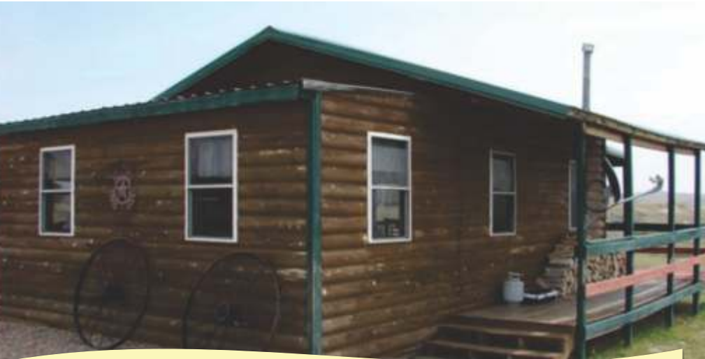
24x20 Cabin w/ bathroom, insulated, bathroom, pine finish inside electric baseboards, 2x12 joices
